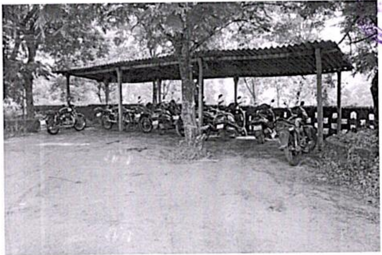
Parking Facility for Staff
