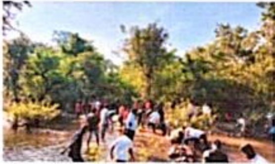
Fig 12: Construction of a small check dam
